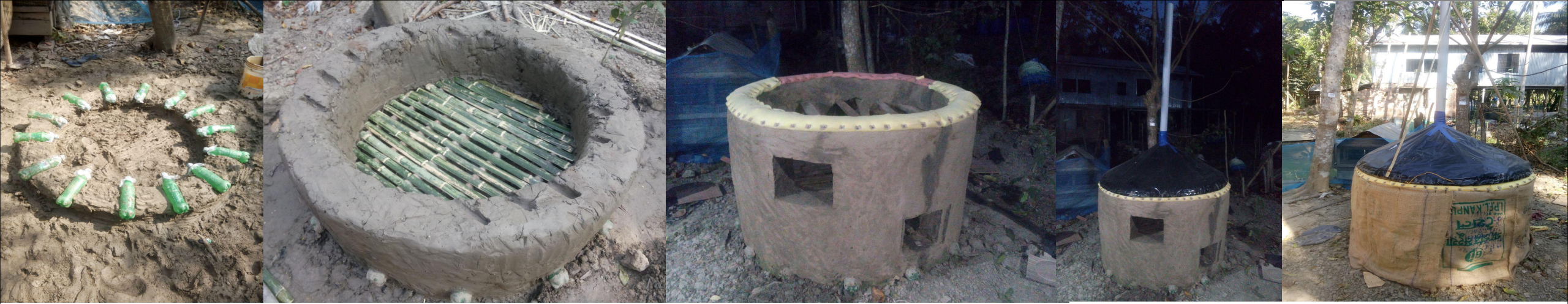
Type A: 1. Make small holes at the bottom of the bottles for circulation of normal air and also tie up the mouth (inside) with mosquito nets to avoid earth worm, snakes, insects to go inside; 2. Place bamboo scaffolding/ platform (layers will be developed); 3. Openings should be like this; 4. Cover the top fixed with a 10ft PVC pipe as a chimney for ventilation of hot air from inside; 5. Cover with sack sprinkled with water for maintaining the mud wall
